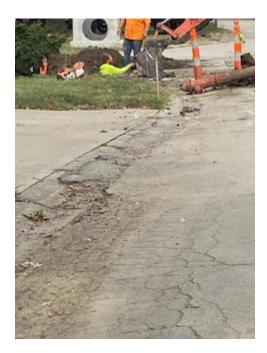
The change order includes a more consistent approach and basically continues a consistent slope from the centerline to the face of curb. Amino has proposed an additional cost of \$24,502.85 for the additional asphalt material.
